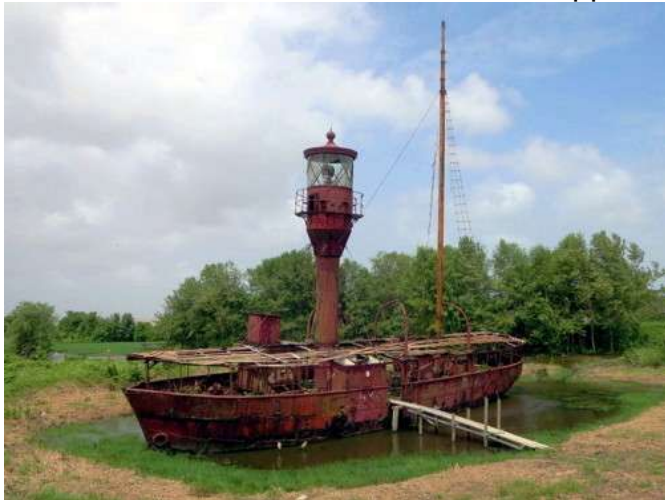
SURINAME - 1, brush cleared away & Access Ramp
