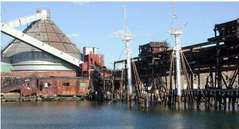
Sunken Lightship No.84 at the Revere Sugar Refinery's abandoned pier in Erie Basin at Red Hook, Brooklyn, NY. Revere Sugar went bankrupt in 1985.
